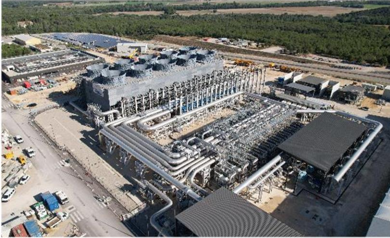
Heat rejection and cooling water system
